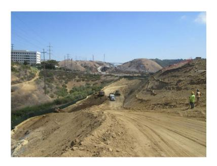
**Photo 1:** Construction activities associated with exporting soil offsite continued during this reporting period. Excavators were observed loading haul trucks to export soil offsite.
