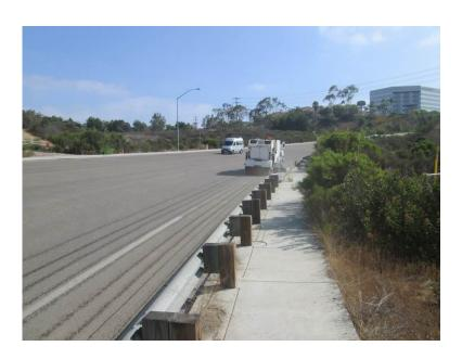
**Photo 3:** In accordance with APM-HYD-1, a street sweeper was observed being utilized along Mira Sorrento Place to remove trac-out.
